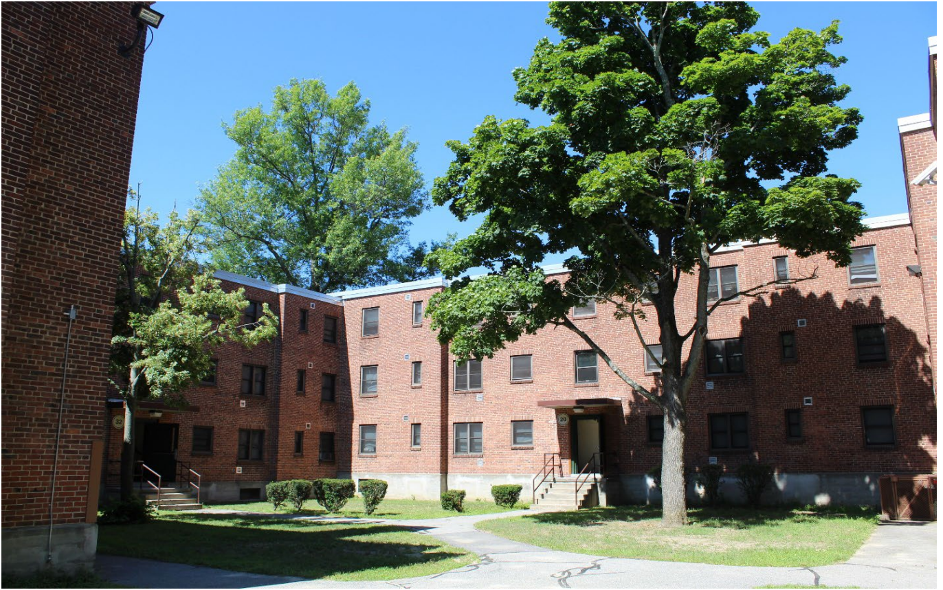
Above and below, current residential buildings at Lakeside Apartments/WHA photos
